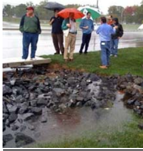
Attendees listen as Underwood and Associates provides a Coastal Plains Outfalls Tour in Anne Arundel County
