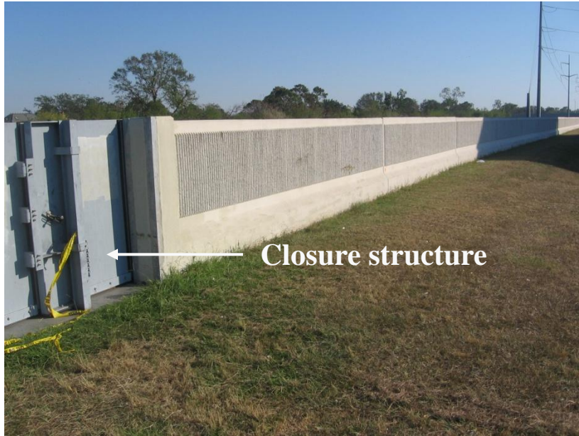
17 th Street Canal Floodwall on top of levee in New Orleans
