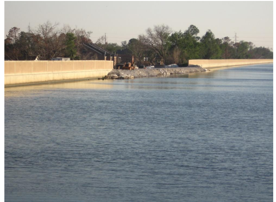
Floodwall Breach- New Orleans
