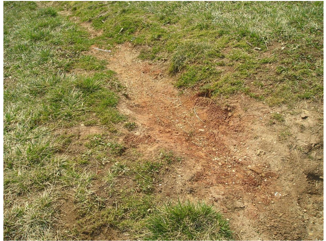
Typical Erosion on the Anacostia Levee
