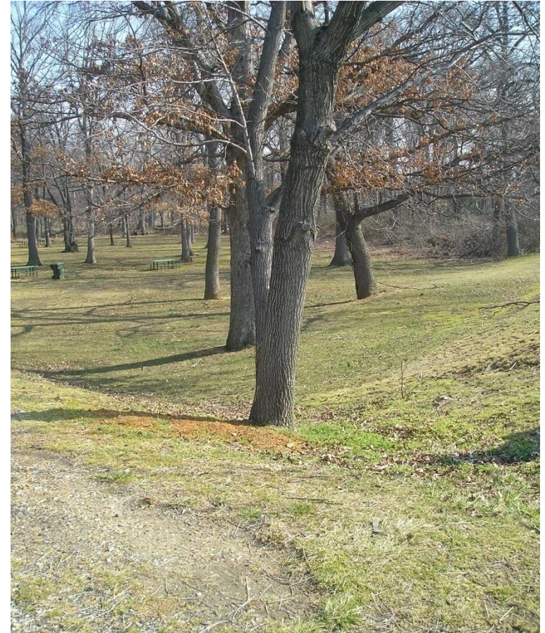
Tree located within 15 feet of the Anacostia Levee System
