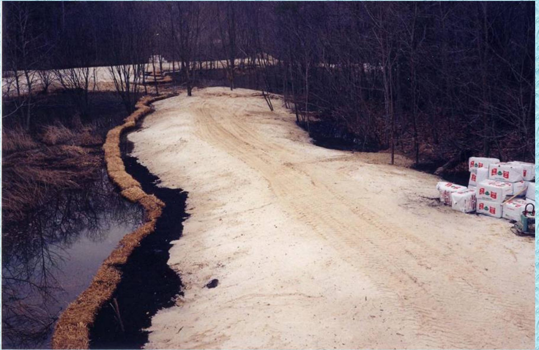
Finished sand berm haul road at Howard's Branch
