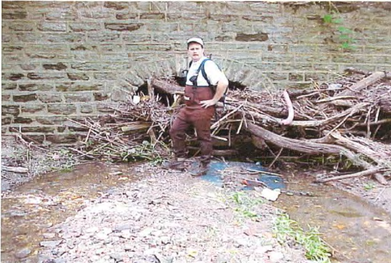
Intake head-wall of culvert (2000)
