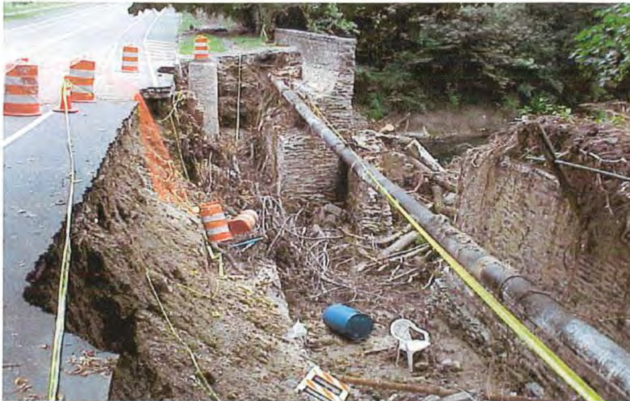
Severe erosion at Haverford Avenue Bridge caused by August 1, 2004 storm
