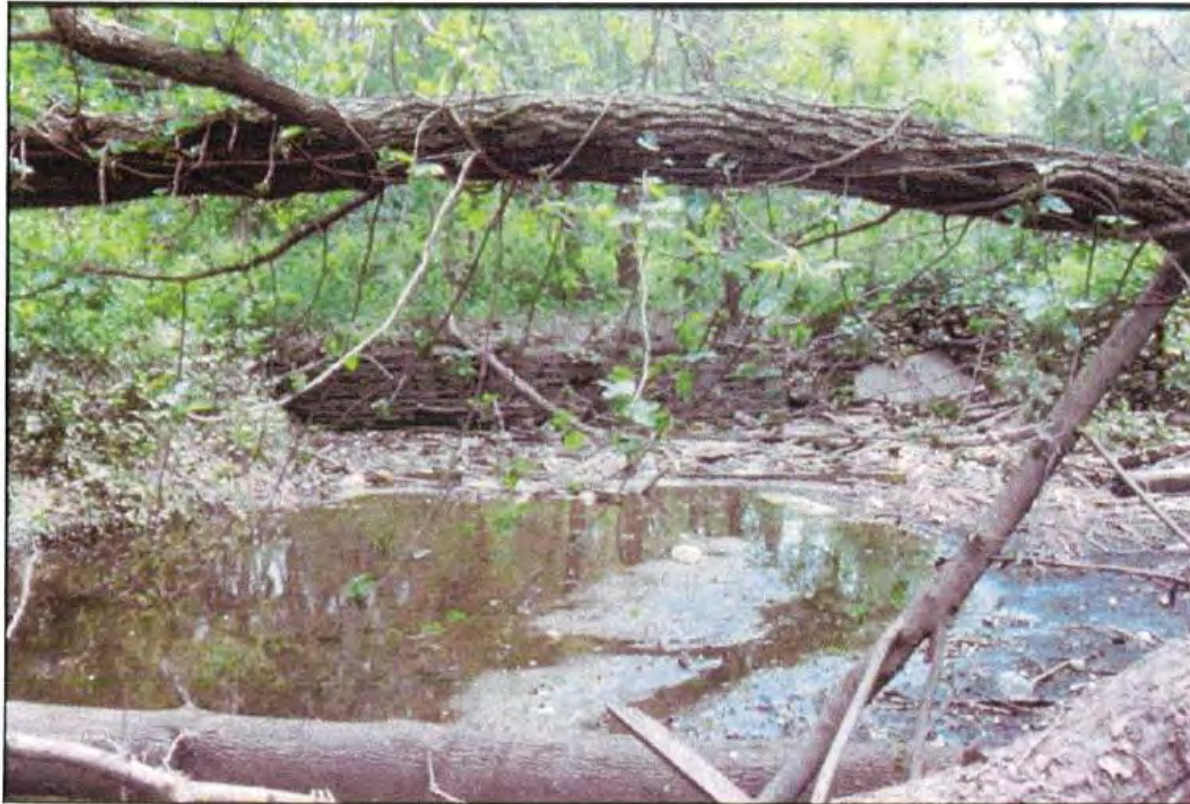
Intake head-wall of culvert (2006)
