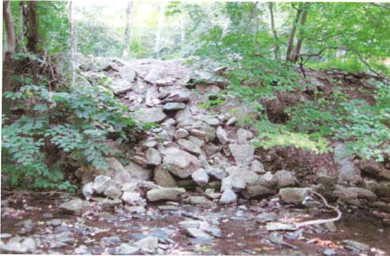
Boulders dumped over slope to repair gully erosion along Reach 1
