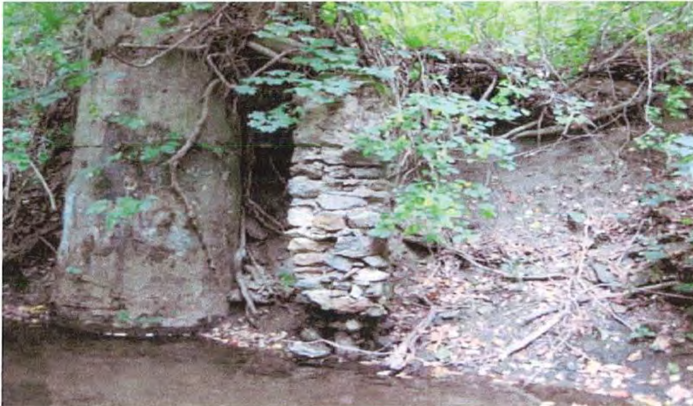
Eroding bank, exposed manhole, old support columns along upstream end of Reach 1
