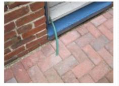
Moisture on the west wall of the basement appears to be from the dehumidifier hose
