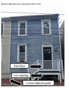
Lowest adjacent grade in this example is the front left corner, the lowest point closest to where the water is coming from. Low opening in this example is the basement window, where water would first enter the building during flooding. First floor opening here is the front door, where the most damage would typically occur if flood waters reached this elevation
