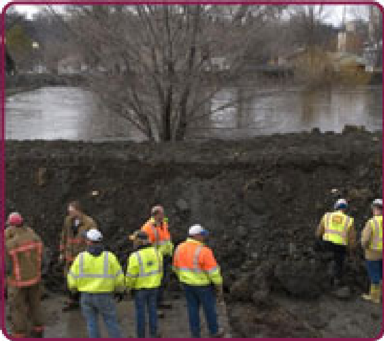
Patsy Lynch/FEMA, National Committee on Levee Safety
