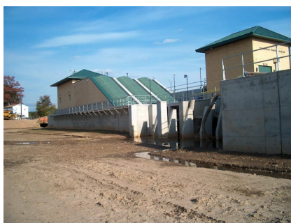
Figure 3 – New Screw Pump Structure and Original Pump House
