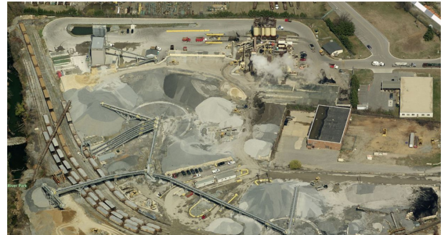
Airgas Facility in Hyattsville, MD Source : Bing Maps
