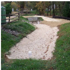
Infiltration Trenches
