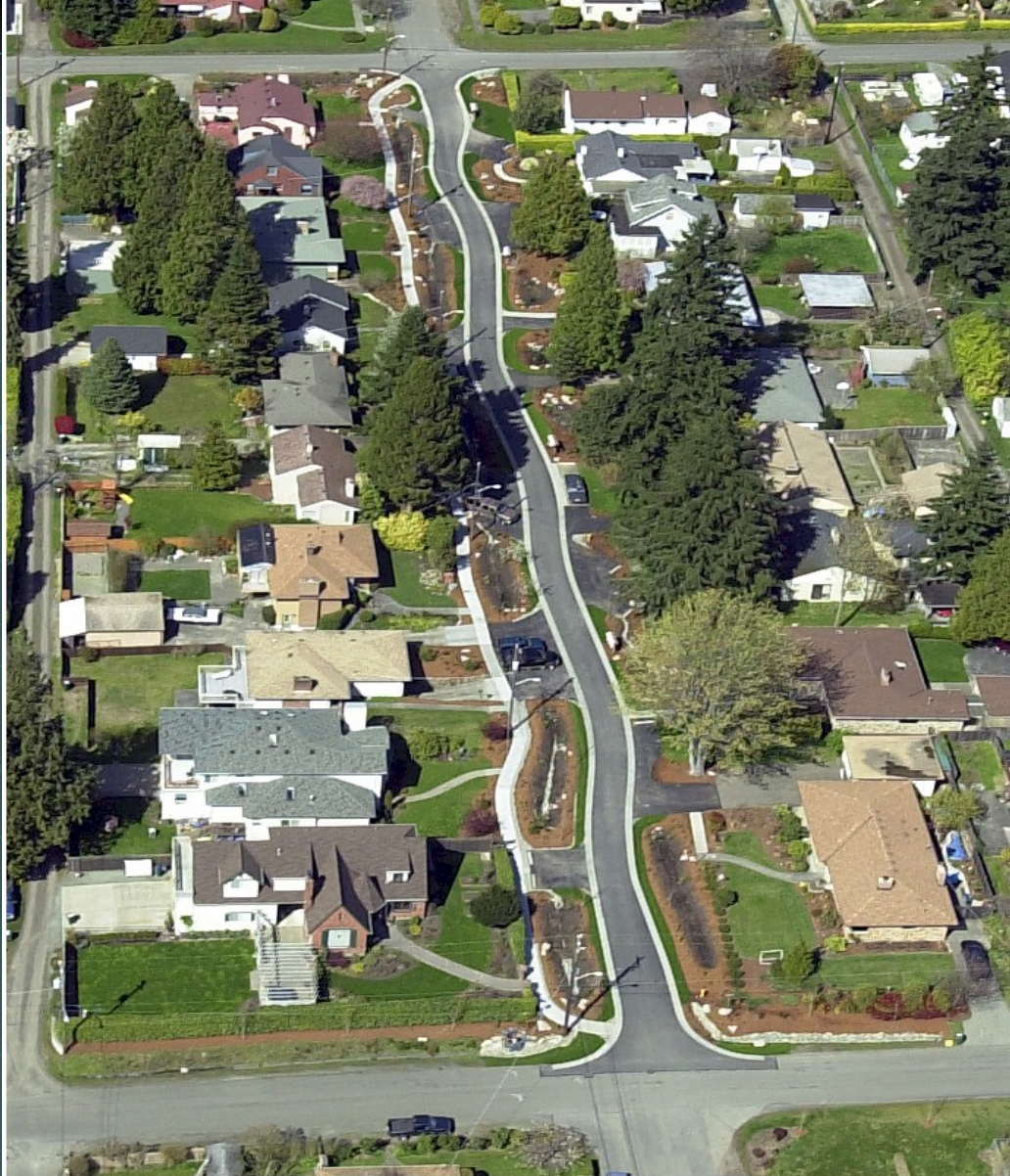
SEA Streets - After Construction 2nd Ave NW - NW 117th St to NW 120th St
