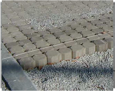
Permeable Interlocking Concrete Pavers (PICP)
