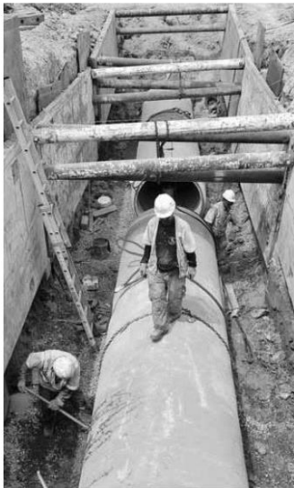
Baltimore Water Pipe
