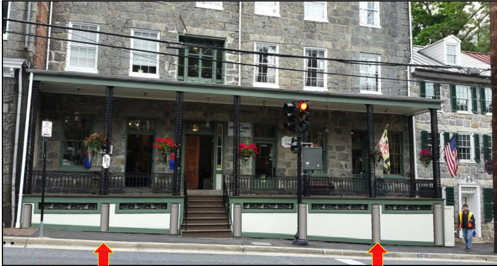
Bollards behind porch
