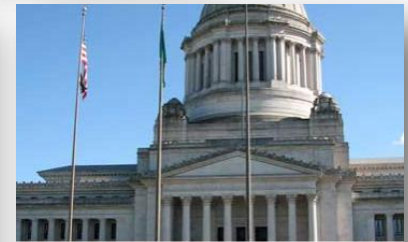
City of Olympia, Washington – Engineered Response to Sea Level Rise
