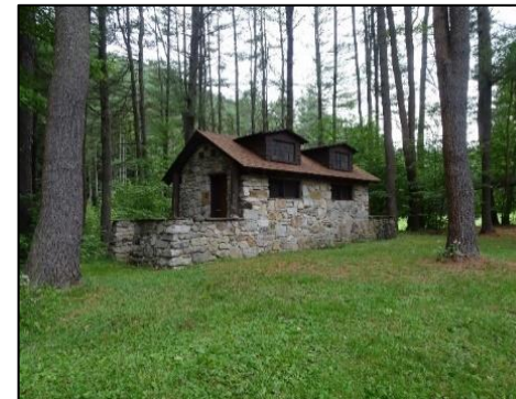
Photo 4: Stone Masonry Building
