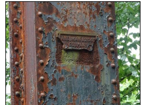
Photo 5: Steel Truss Bridge
