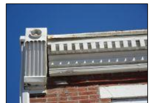
Photo 10: Brackets & Dentil Molding
