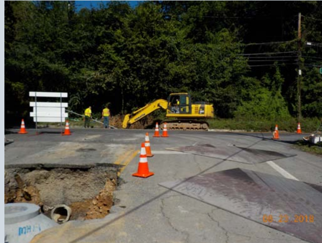
Milnor Avenue MH_1-1 Manhole to New I_1-1 Inlet for US 220 Culvert Crossing. Crossing depth 11.75 feet under 20" water main line
