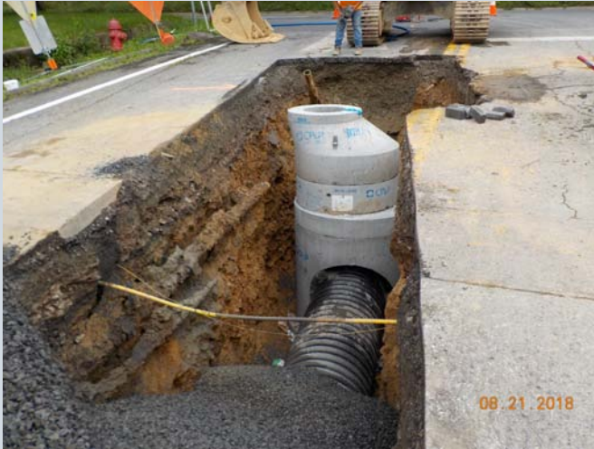
Milnor Avenue New MH_1-1 Manhole Approx. 12.5 Foot Depth
