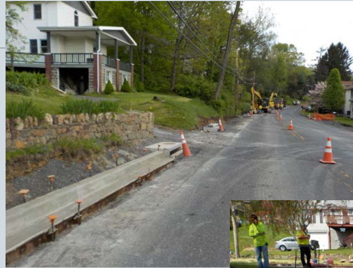
Aspen Avenue New I_4-3 Inlet Modified SHA COG Inlet Approx. 11 Foot Depth
